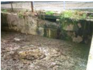
Scum and crust formation before application of Advetec 900.
